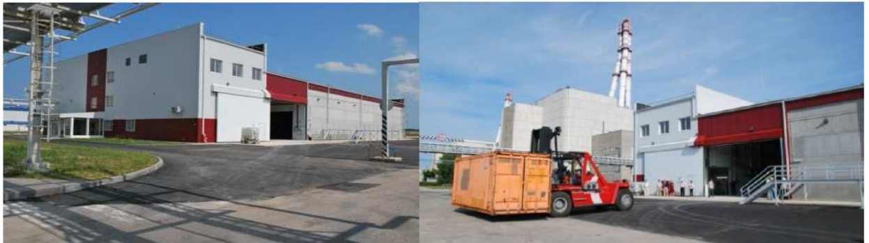
Fig. 14. Buffer Storage building
