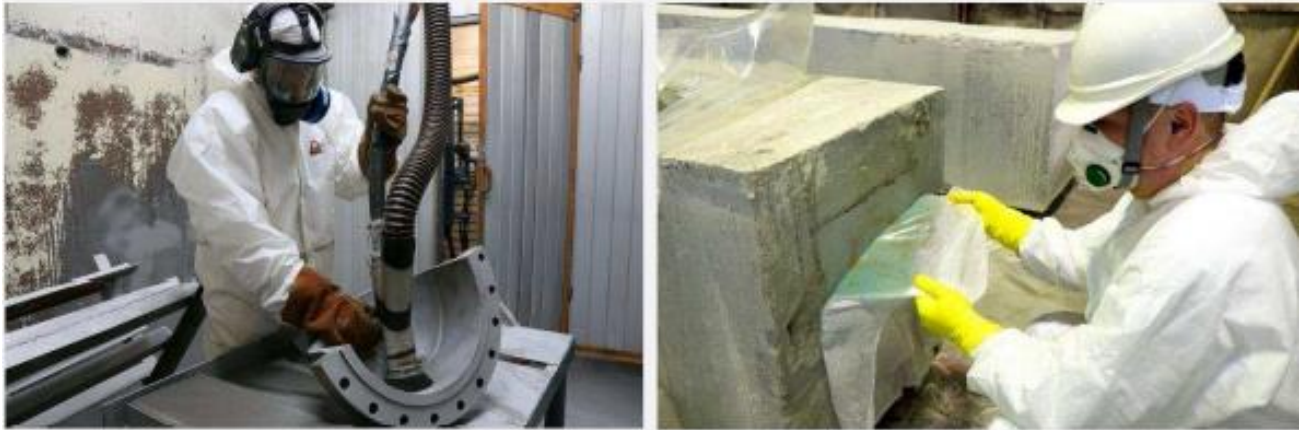
Figure 19. Decontamination methods: • physical (mechanical) techniques such as blasting, jetting, wiping, brushing, etc; • ultrasonic techniques; • chemical techniques
