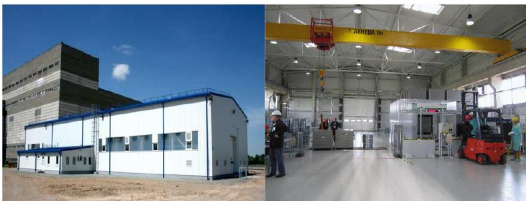
Fig. 17. Pictures of operated Free Release measurement Facility 1.2. Short Description of the Project
