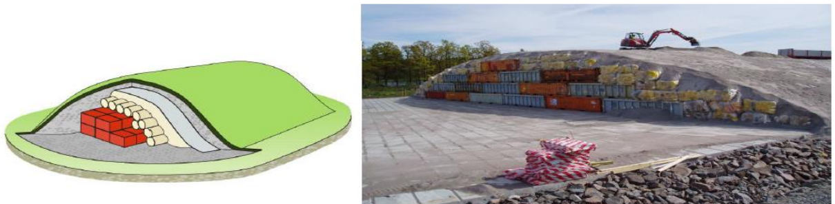
Fig. 15. Conceptual view of waste loading in the designed Repository for Short-Lived Very Low Level Waste and picture of operating Sweedish Oskarshamn NPP Repository
