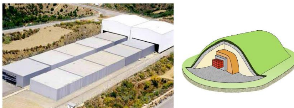
Fig. 16. Conceptual view of the Near Surface Repository, waste loading diagram
