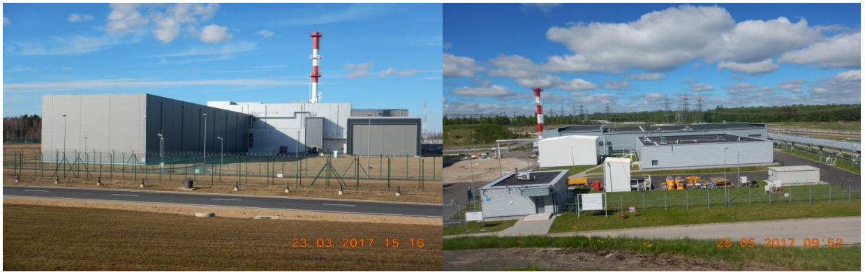
Fig. 13. General view of SWRF and SWTSF under construction
