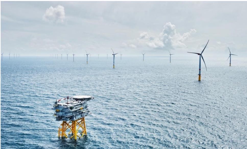
Figure 7. Example of substation design with jacket foundation.
