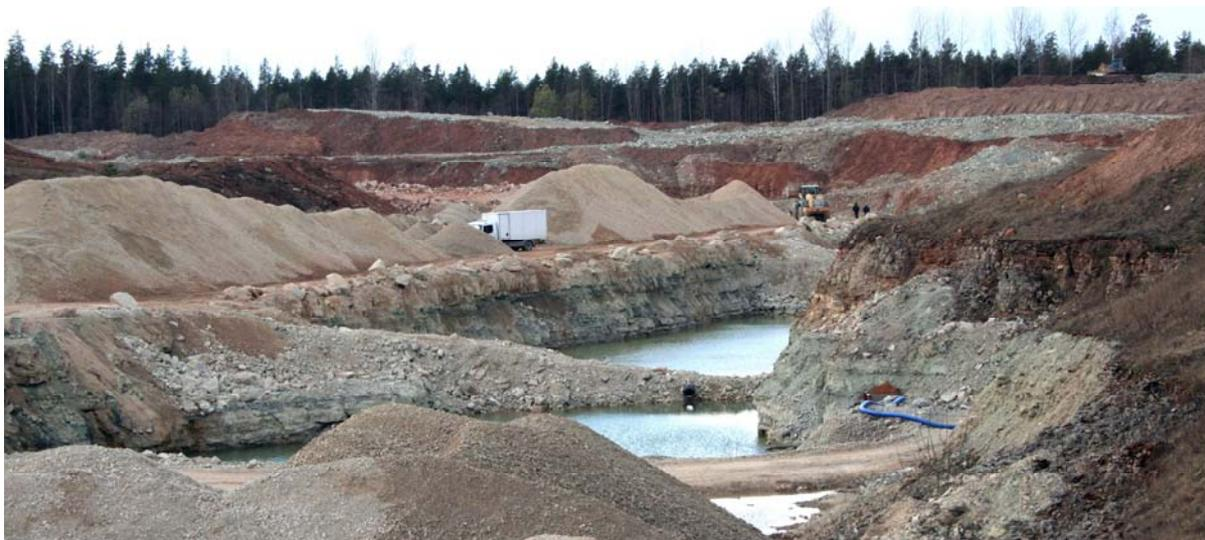
Figure 16. Ape quarry in April 2014. Despite the fact that the dolostone is covered by a thick clay layer, the sedimentation basins in the quarry allow to pump out water which content of suspended solids is low.
