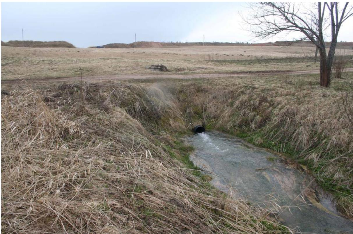
Figure 14. The end of the outlet pipe that flows from Ape quarry to the outlet ditch. The diameter of the pipe is about 30 cm. Off in the distance are embankments of quarry overburden. Sample for general water analysis was taken 14 April 2014 directly from the outflow.
