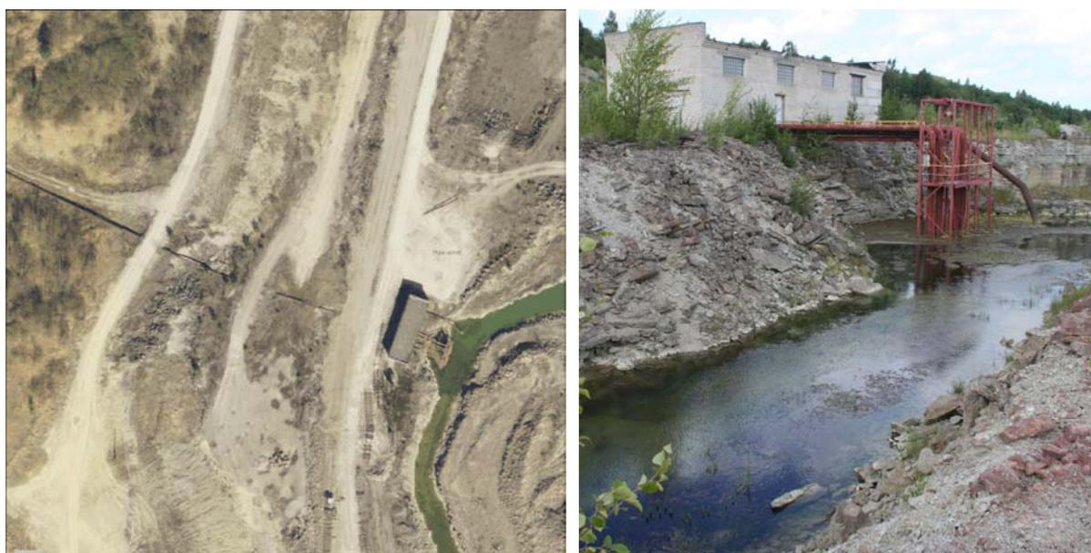
Figure 7. Pumping out water from the approx. 1.5 km<sup>2</sup> Aru-Lõuna cement limestone quarry. The amount of water pumped out of Aru-Lõuna quarry can be as much as 400 litres per second. Water collector ditch, other ditches, pump station and pipeline as seen on orthophotograph (left) and photograph (right).
