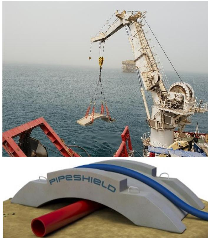
Figure 3.19. Method for constructing and laying concrete structures on a cable line (source: [www.pipeshield.com/products/concrete-structures](http://www.pipeshield.com/products/concrete-structures))
