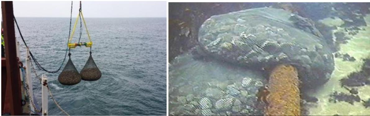
Figure 3.18. Method for constructing and laying rock bags on a cable line (source: [www.bluemont.com.au/erosion/kyowa-rock-filter-bags/offshore-subsea](http://www.bluemont.com.au/erosion/kyowa-rock-filter-bags/offshore-subsea))
