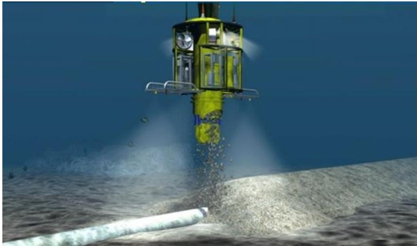
Figure 3.17. Visualisation of a rock dump construction (source: [www.offshore-fleet.com/data/rock-dumping-vessel.htm](http://www.offshore-fleet.com/data/rock-dumping-vessel.htm))
