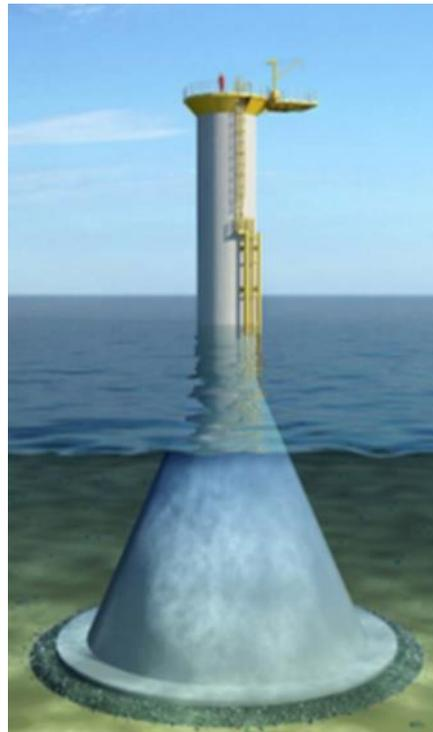
Figure 3.7. Example of a gravity-based structure (source: Ramboll)
