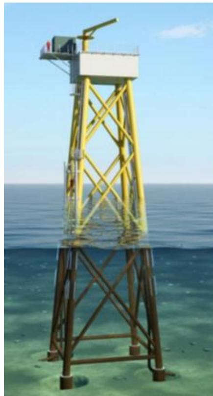
Figure 3.6. Example of a piled jacket foundation (source: Ramboll)
