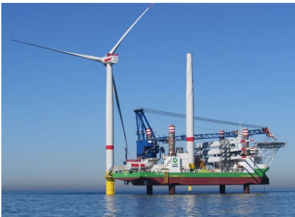
Figure 15. Assembly of wind turbines with a jack-up vessel. Source: COWI.
