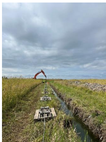
Photograph 4. Installation of the second 110 kV submarine cable of the Väike Väin strait on the coast of Muhu using the open method (Skepast & Puhkim OÜ, 21.08.2024)
