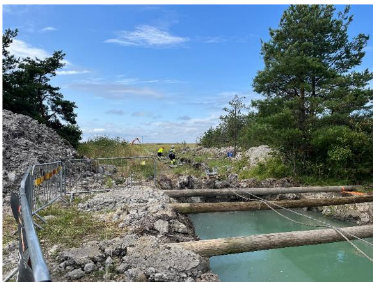
Photograph 4. Installation of the second 110 kV submarine cable of the Väike Väin strait on the coast of Muhu using the open method (Skepast & Puhkim OÜ, 21.08.2024)
