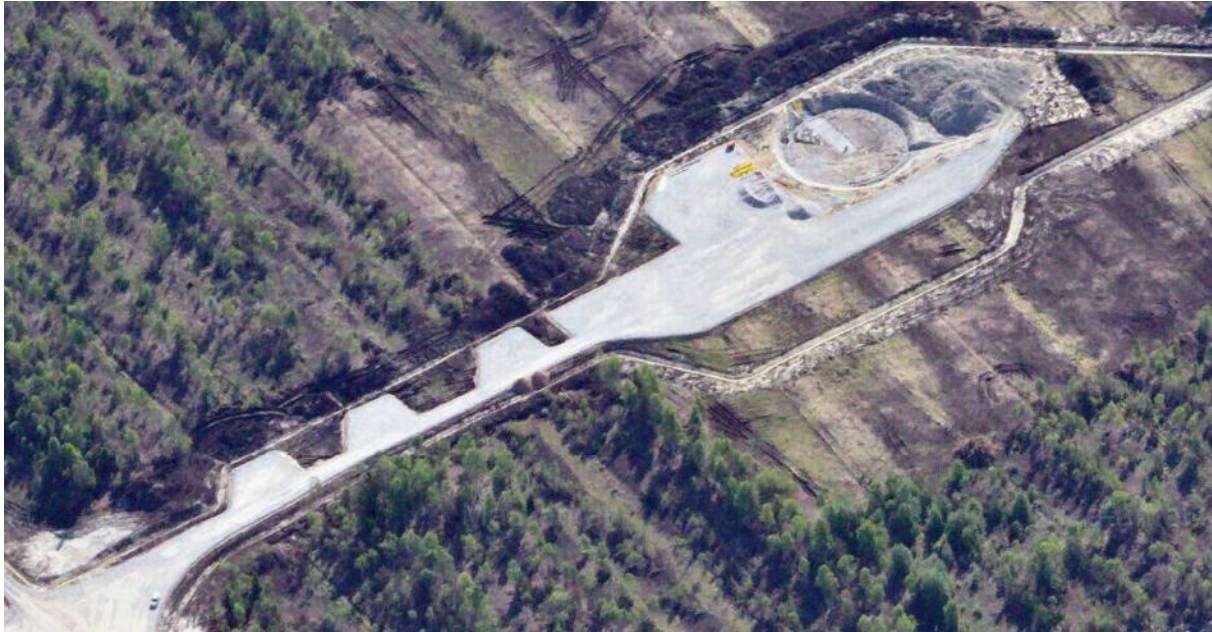
Figure5 . Possible wind turbine foundation area with assembly sites. Source: Land Board aerial photograph – Tootsi/Sopi wind farm. The exact shape and area of the assembly site depends on the specifications of the wind turbine manufacturer.
