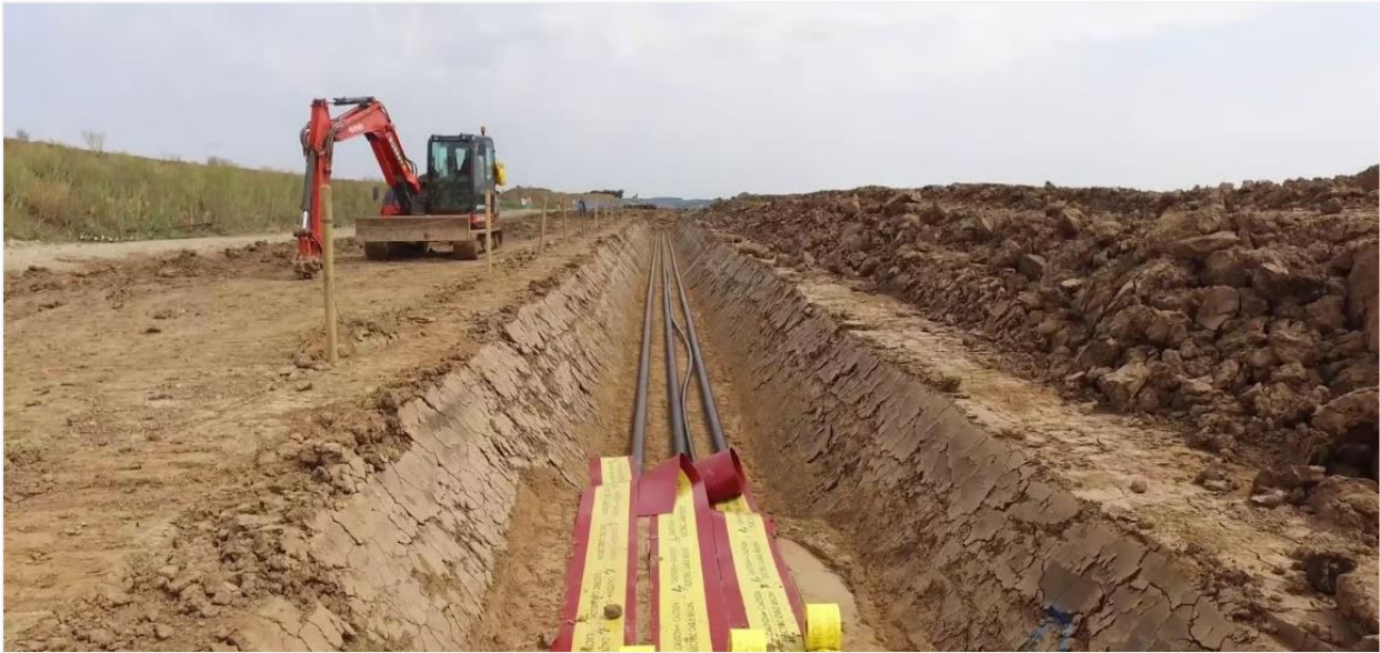
Fig. 2.2.19. Cable laying using the open-trench method.
