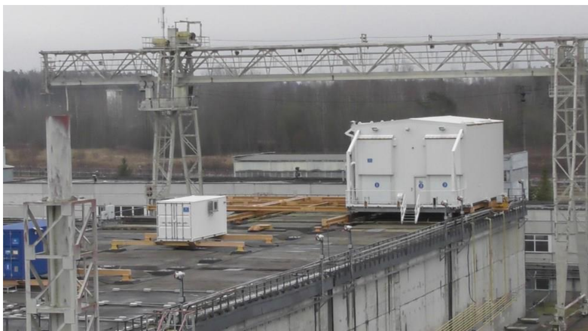
Figure 3.2-5. INPP operational SRW storage building No. 157/1 with group G1 and G2 SRW retrieval unit RU-2
