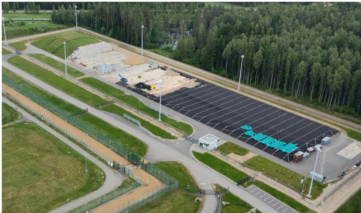
Figure 3.2-29. VLLW repository module with engineering barriers and protective wall formed after a particular loading campaign
