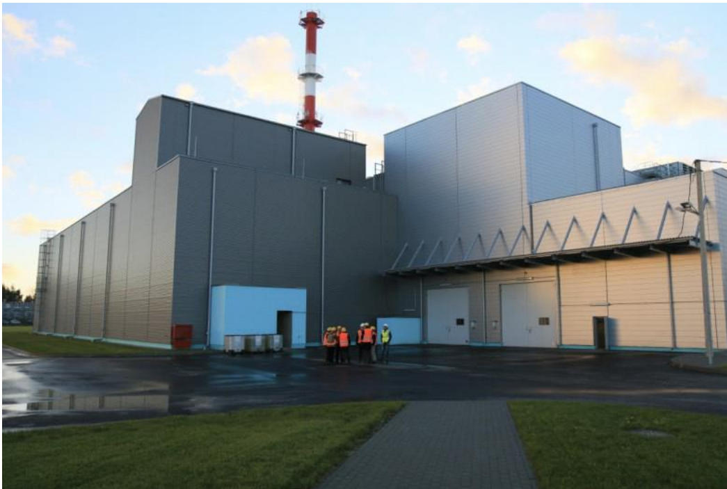
Figure 3.2-22. INPP Solid Radioactive Waste Treatment and Storage Facility (SWTSF)
