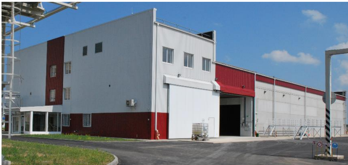
Figure 3.2-26. The building of the VLLW repository buffer storage facility
