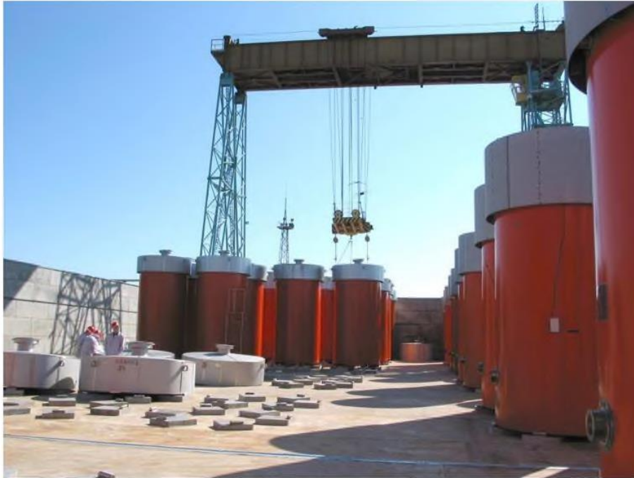
Figure 3.2-1. SNF storage facility ISFSF-1 with casks
